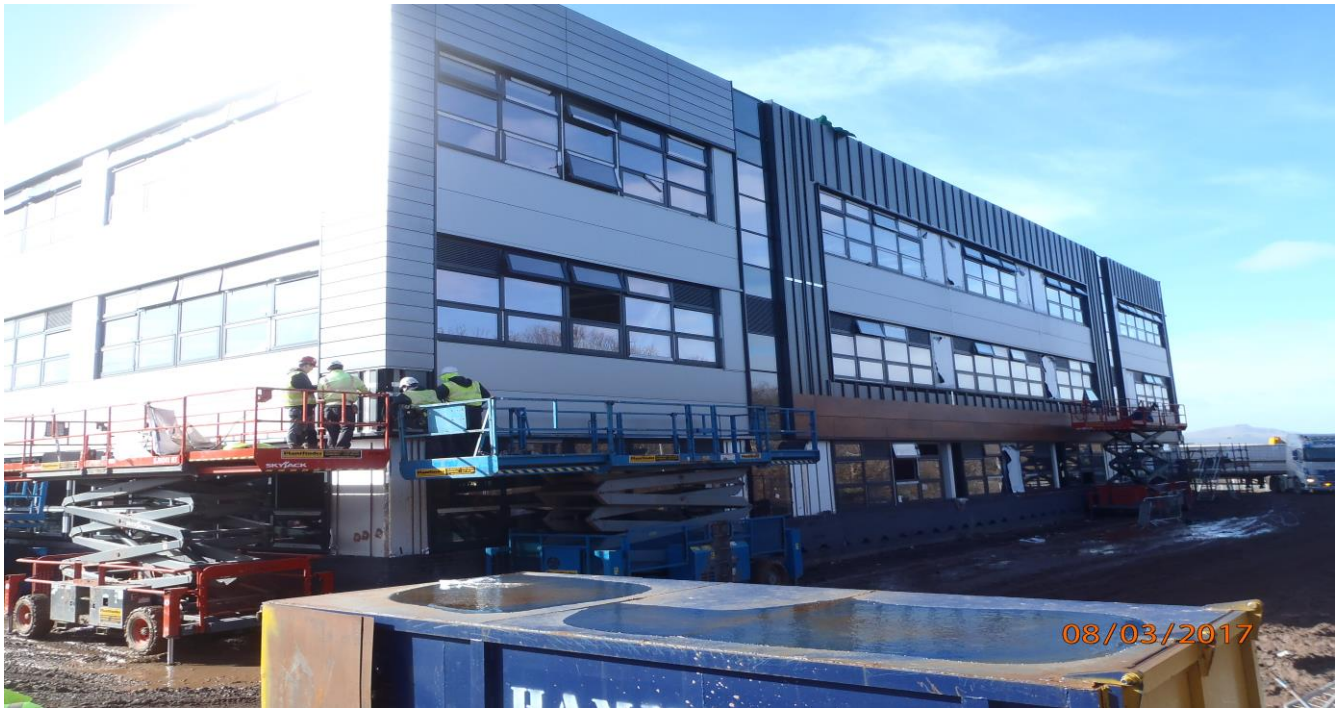
Installation of Timber Cladding to Teaching Block
