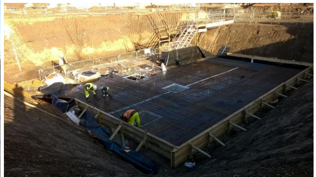
'Swimming Pool Structure Being Formed'
