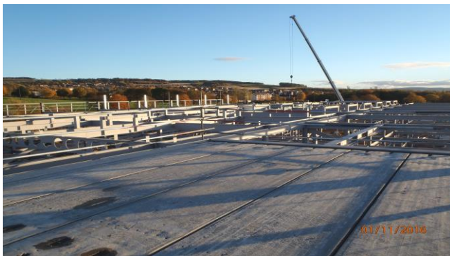
'Pre Cast Concrete Floor Units'
